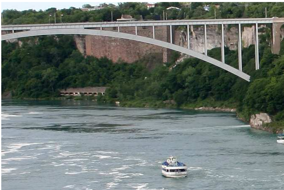
Obr. 1.4.: Ruiny hydroelektrárny Schoellkopf Power Station No. 3
